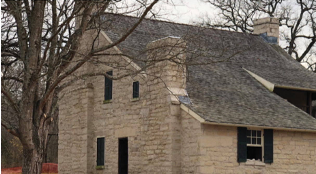
Hays House renovation
